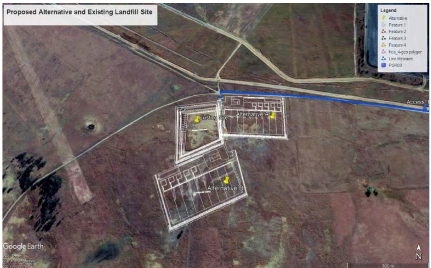
Figure 2.1: Existing landfill site with the alternatives of the proposed new general waste disposal site.
