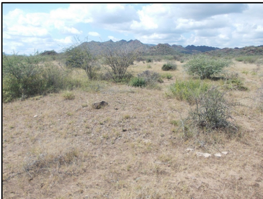
Figure 6: View of historical foundation
