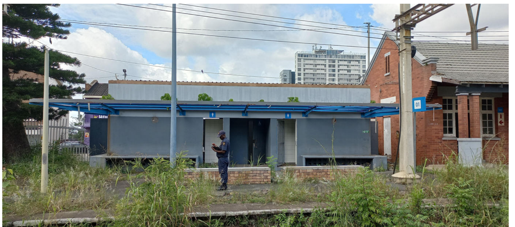
6. EXISTING PUBLIC ABLUTION BUILDING
