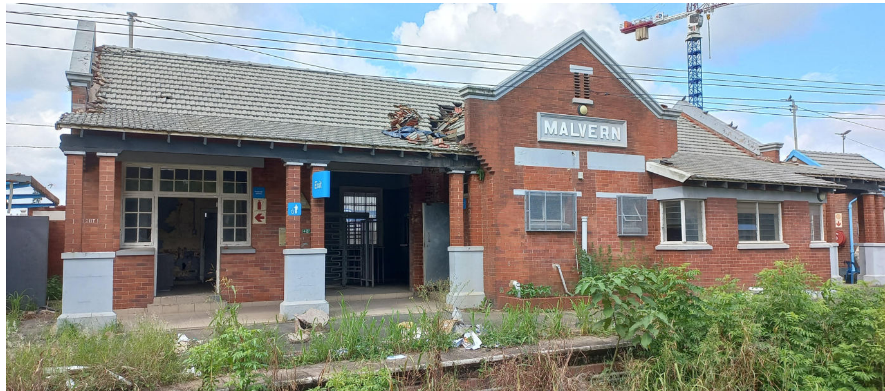
5. EXISTING STATION BUILDING - EXTERNAL
