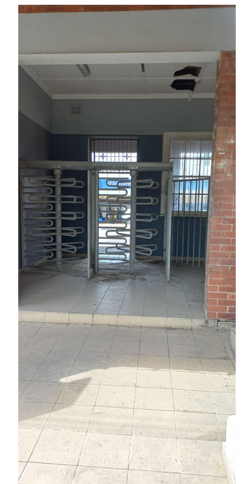
4. EXISTING PUBLIC ENTRANCE
