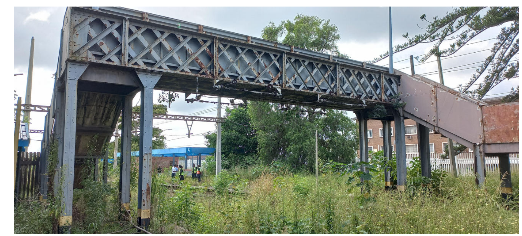
8. EXISTING PUBLIC PEDESTRIAN BRIDGE
