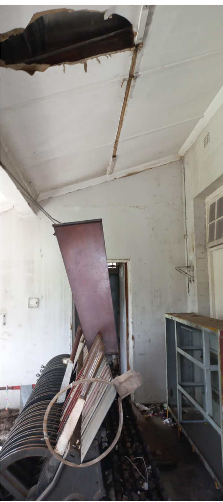
2. EXISTING STATION BUILDING - INTERNAL
