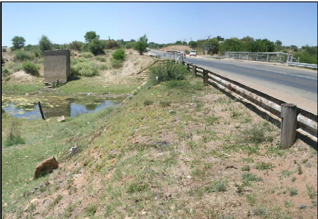
Photo 3: View of bridge crossing the Harts River at Schweizer-Reneke. The pipelines will be attached to the bridge.
