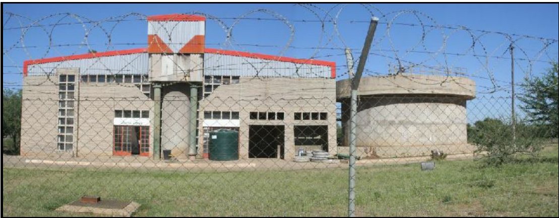
Photo 2: Bloemhof Water Treatment Works (WTW).
