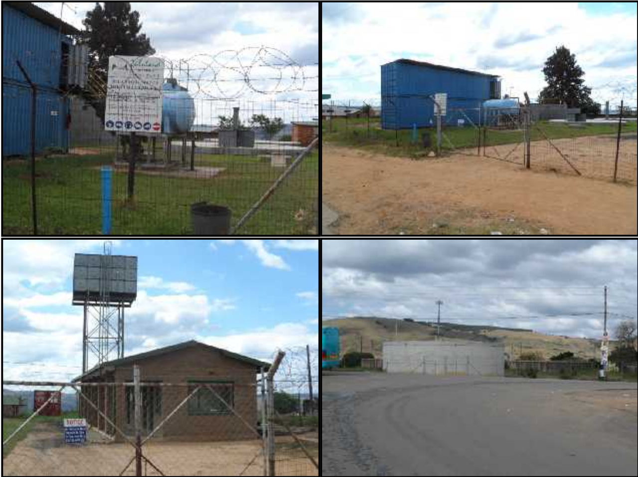
Figure 4 – Existing water treatment and distribution plant
