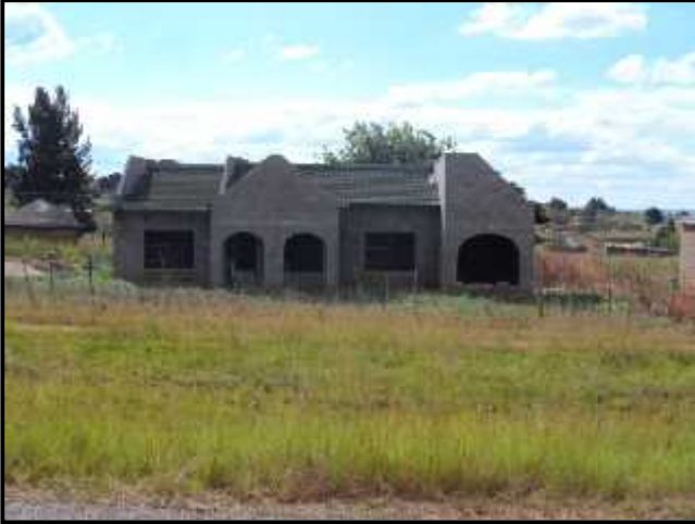
Figure 9- Example of modest house under construction
