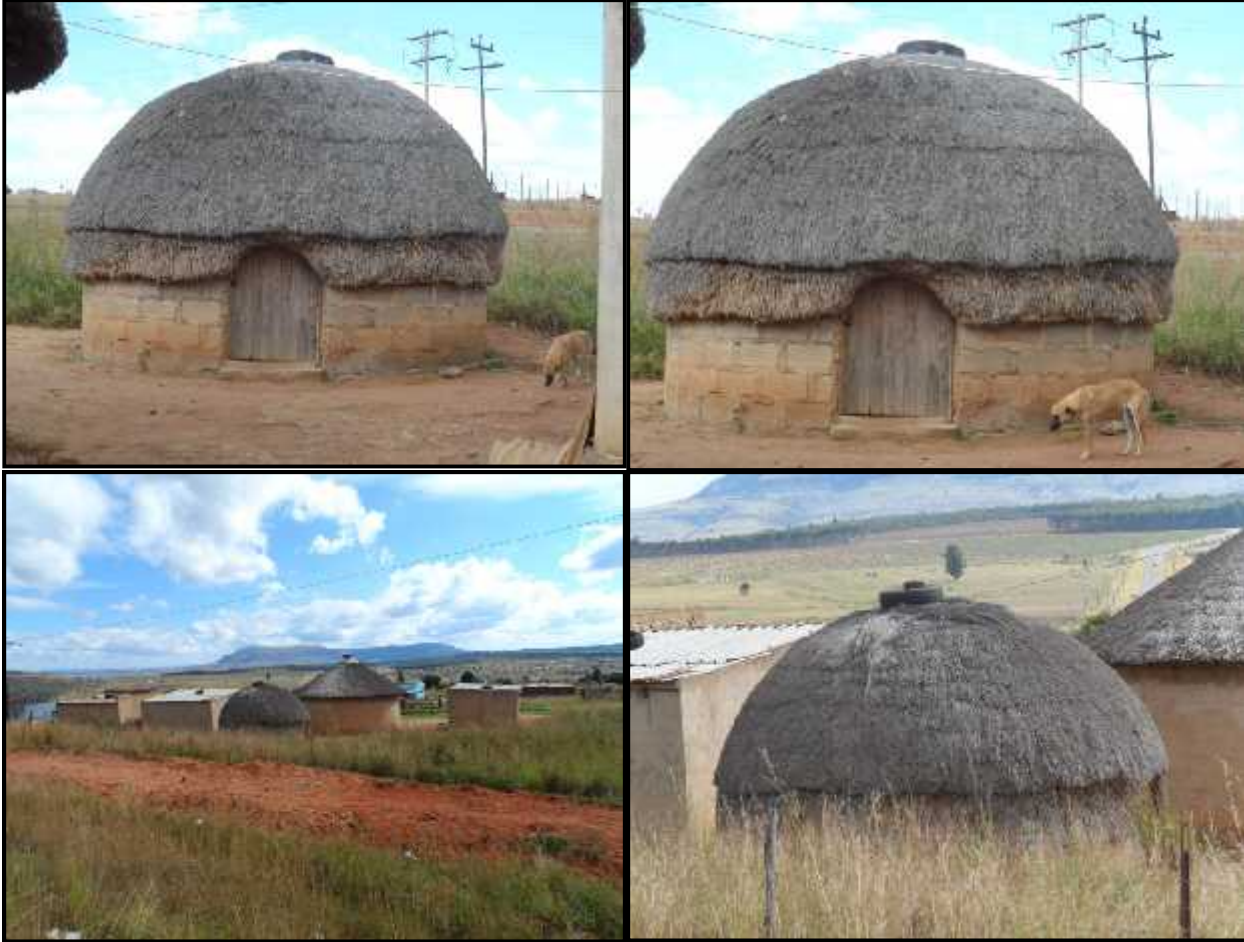
Figure 6 - Example of village homestead consisting three flat roofed houses, a modern rondaval and modernised beehive structure
