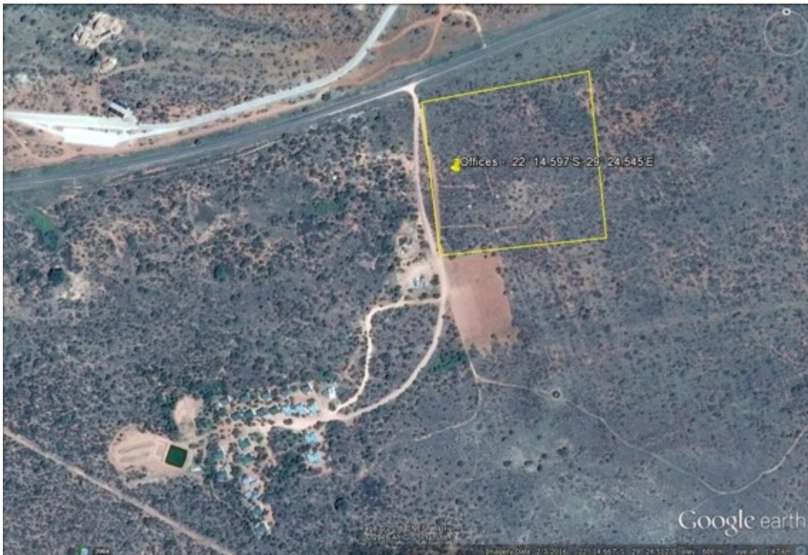
Plate 1: Google Earth Image of the Proposed Office Complex site opposite the Mapungubwe Interpretation Centre (Courtesy: SanParks) (see Appendix 1 for architectural plans)
