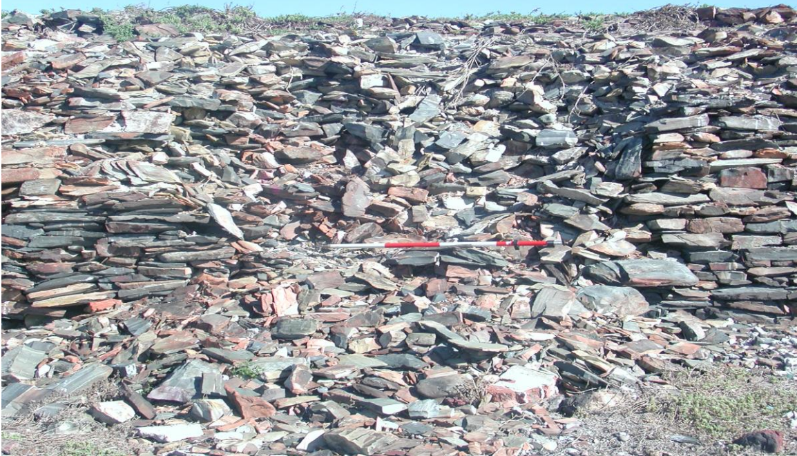
A 2.5 m long collapse separates façade 2j from 2i.
