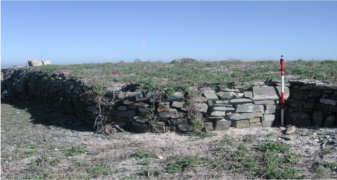
Intersection of walls 1 and 2
