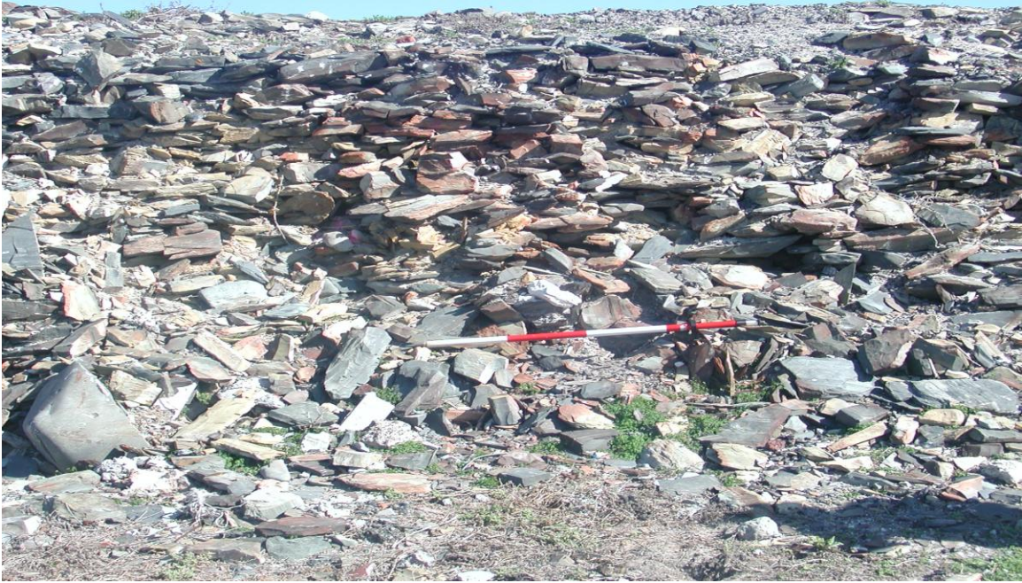
FA 4 m long collapse separates façade 2h from 2i.
