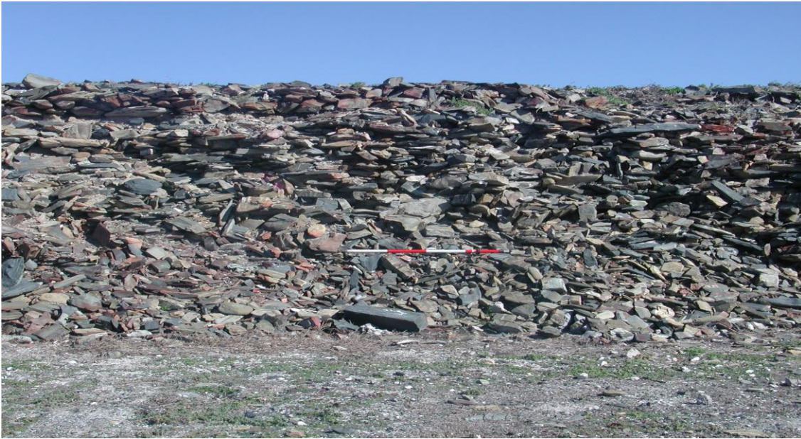
A 5.5m long collapse separates façade 2j from 2k.
