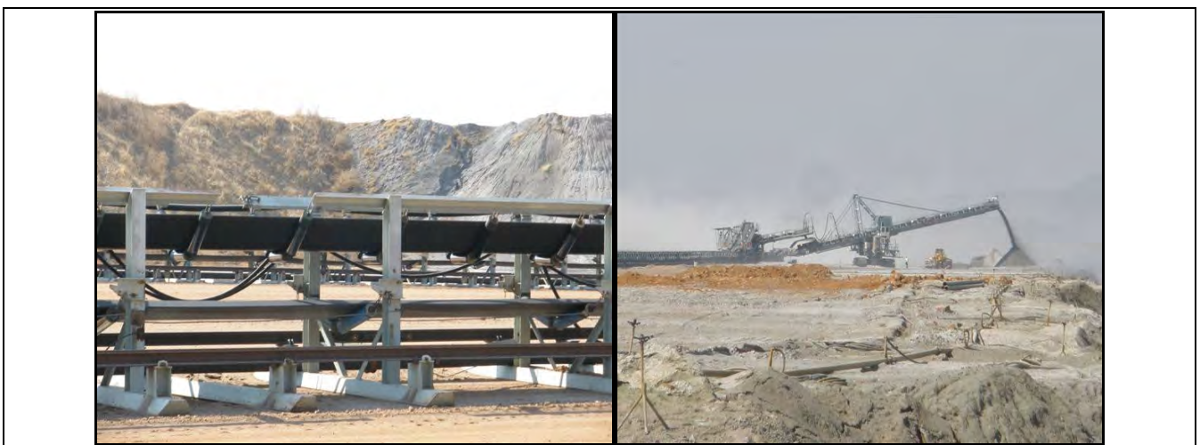
Ash is transported with a conveyor belt from the power station to the ash disposal facility
