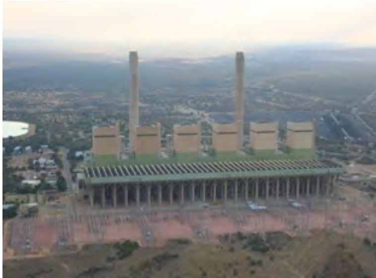
Figure 1: Matimba Power Station
