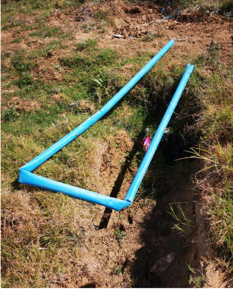
Figure 15 Exposed water pipeline repaired
