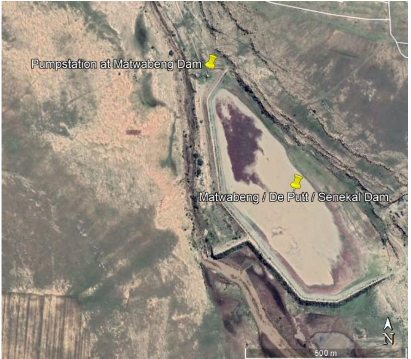
Figure 7 De Put / Matwabeng / Sekekal off-channel storage dam
