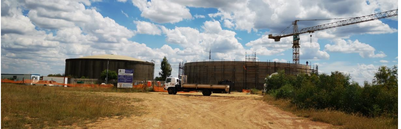
Figure 12 11 Ml Reservoir under construction
