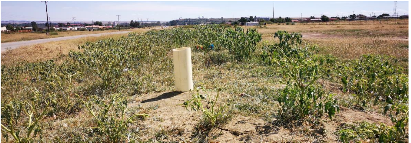
Figure 24 Manhole for gravity under construction
