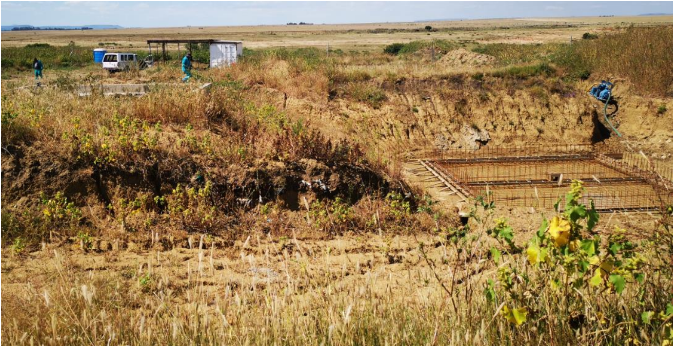
Figure 23 Sewer sump and pumpstation under construction
