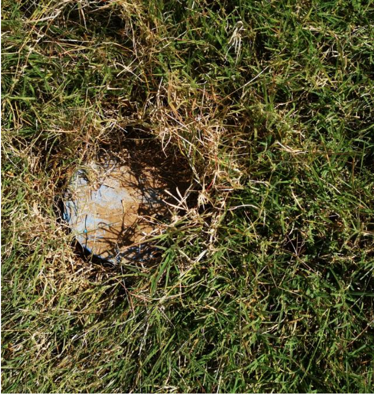
Figure 17 Water valve onsite 28°20'46.56"S 27°38'17.38"E
