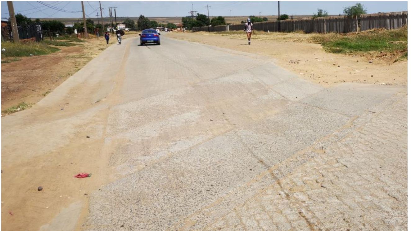
Figure 27 Block paved main street access
