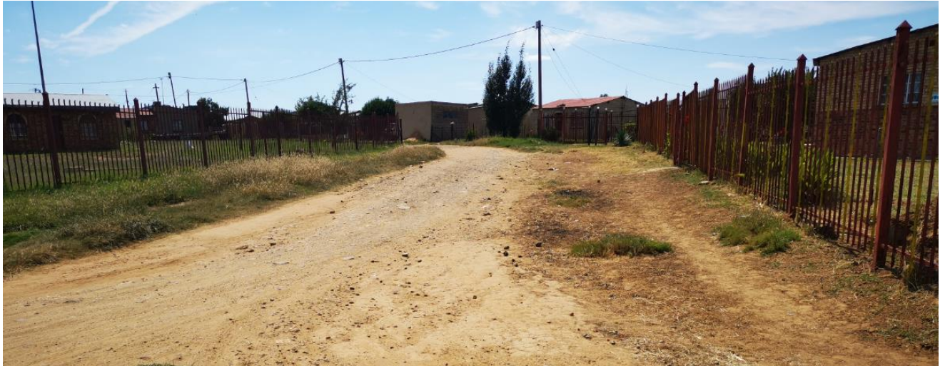
Figure 26 Gravel road internal street
