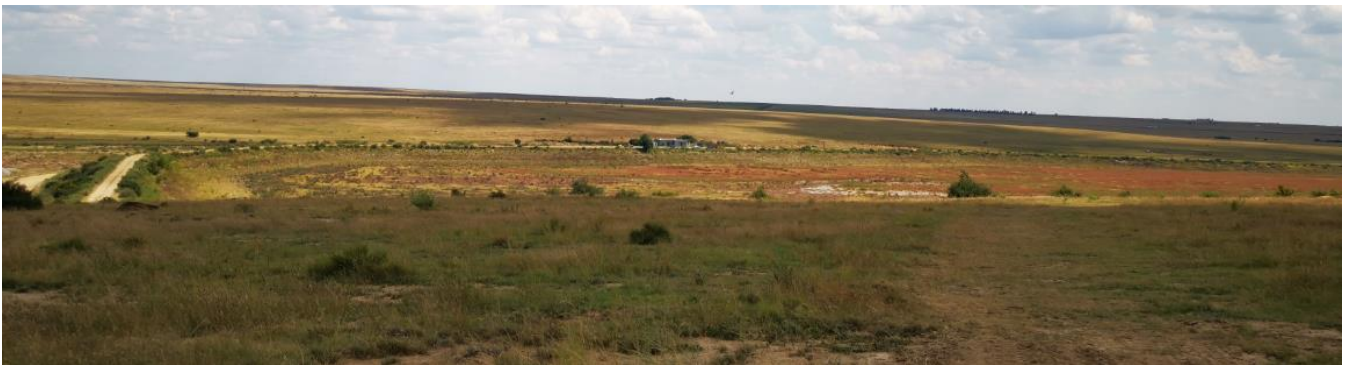
Figure 8 De Put / Matwabeng / Sekekal off-channel storage dam view
