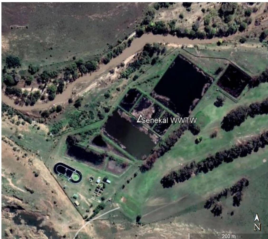
Figure 21 WasteWater Treatment Works (WWTW)
