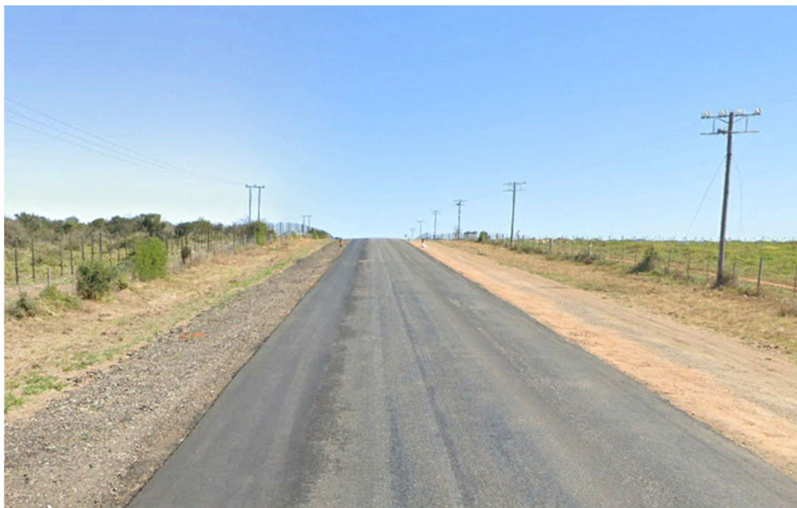
Figure 4-14: View from farm access on R75 in a north-western direction (Source: Google Earth Pro)
