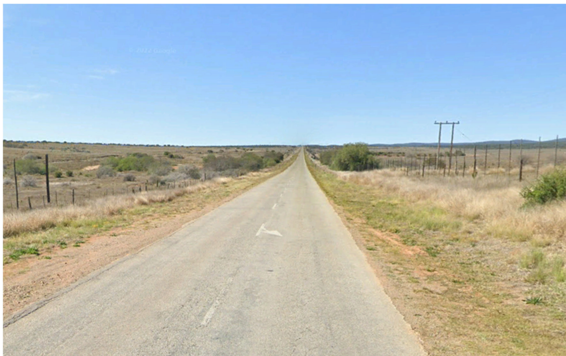
Figure 4-12: View from intersection of R75 / MN50455 in a south-eastern direction (in R75)
