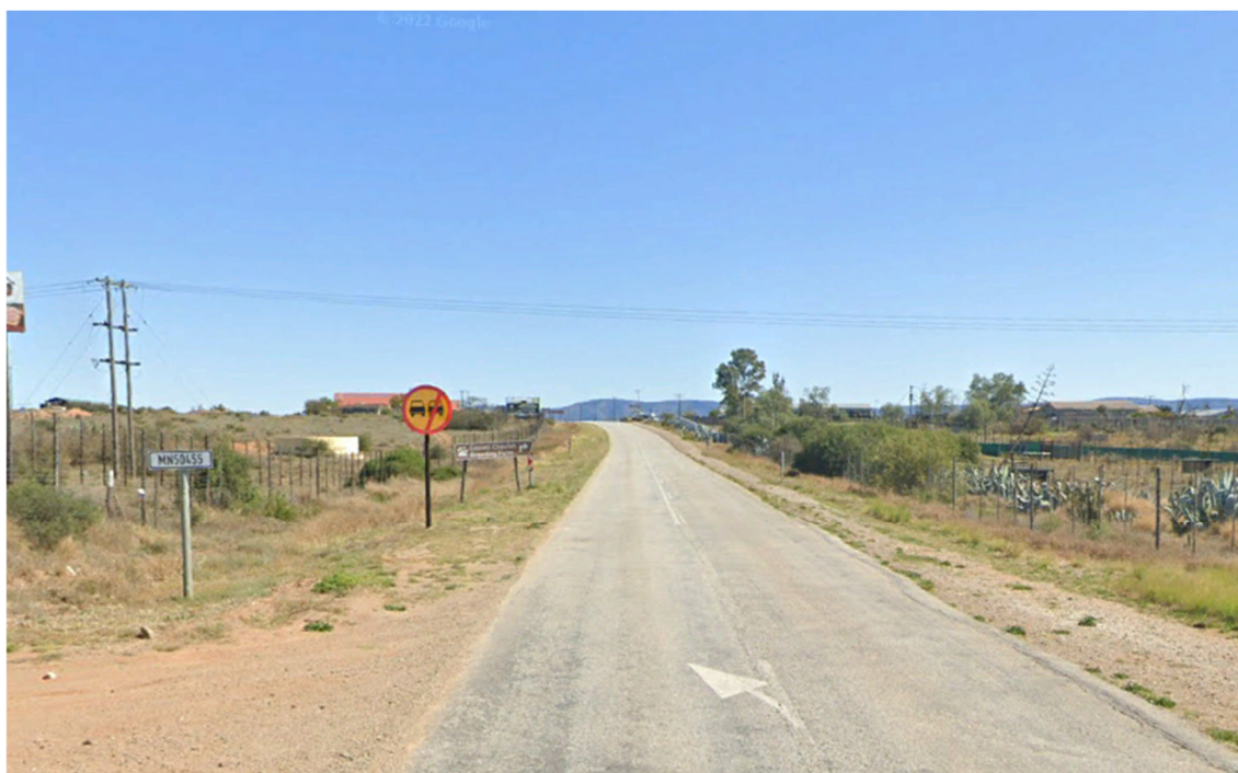
Figure 4-11: View from intersection of R75 / MN50455 in a north-western direction (on R75)
