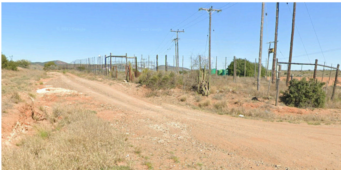
Figure 4-6: MN50455 towards Skilpad Substation
