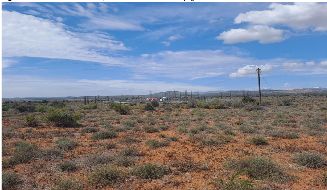
Figure 1.2: Location of the Skilpad Substation on the Mayogi Farm
