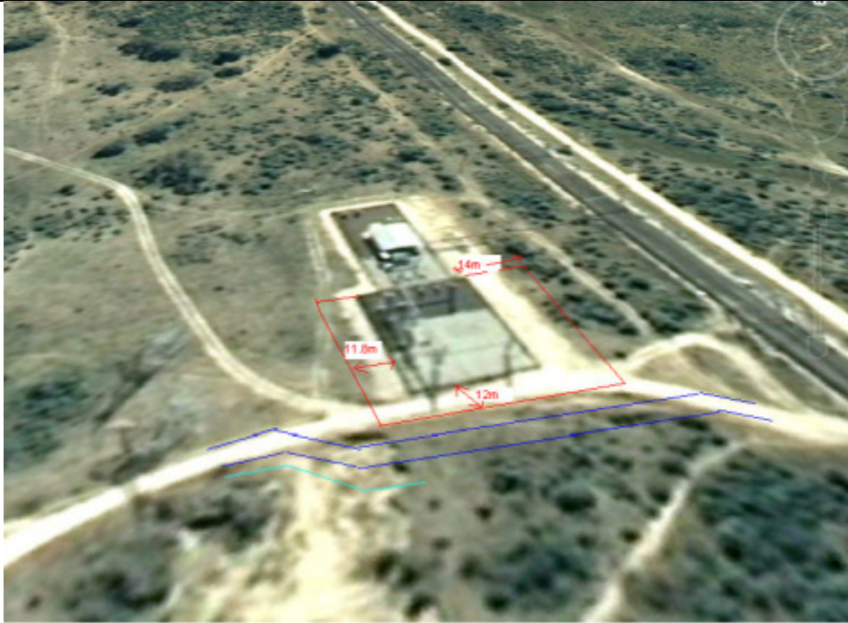
Figure 6: Mbumbu substation footprint expansion
