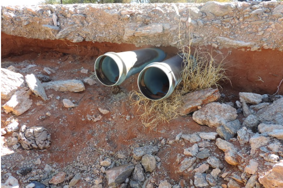
Figure 6 Hardpan carbonate material (underlying the Coega soil form) has been used to stabilise the sandy red apedal soil where farm roads crossed over preferential flow paths
