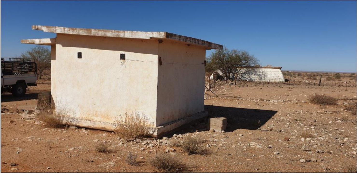
Figures 6.15 Store room or machine room associated with the historic tungsten mine (Pt 21)
