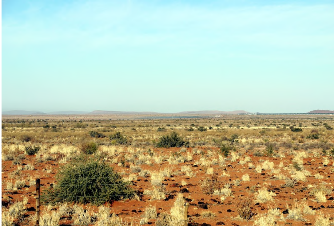
Plate 6, View of Sirius Solar PV Project One, currently under construction (centre picture) from the Lutzputs Road.
