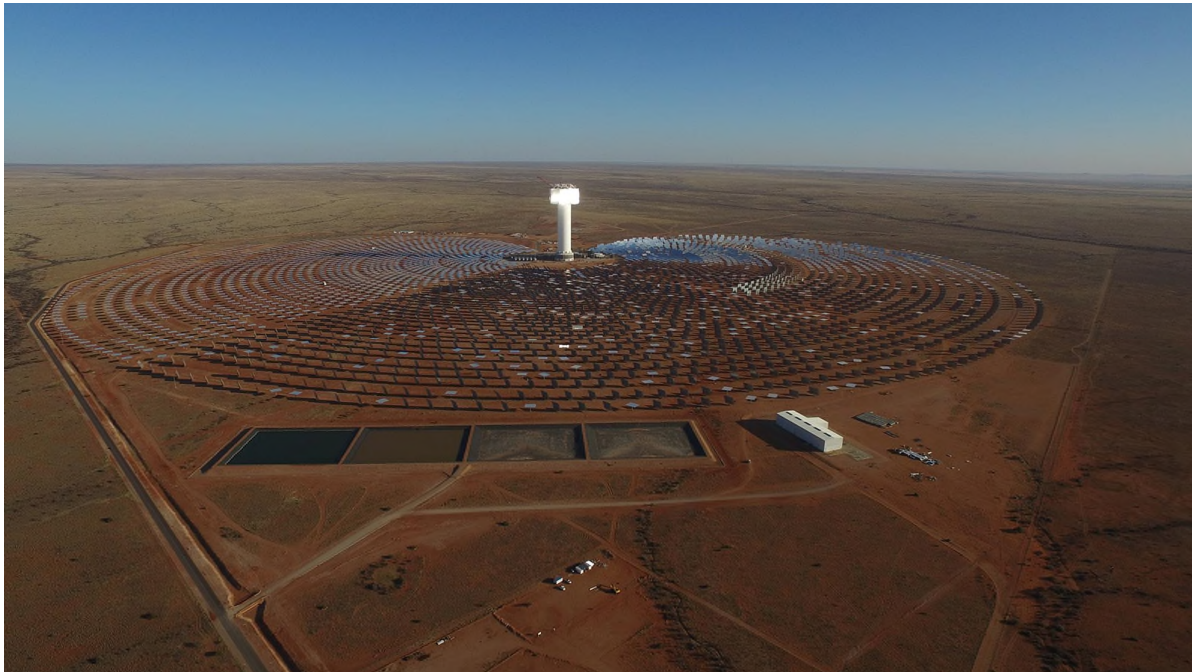
Figure 4.3: Operational Khi Solar One located in the southern corner of Portion 3 of the Farm McTaggarts Camp No. 453 (source: www.energy.org.za )
