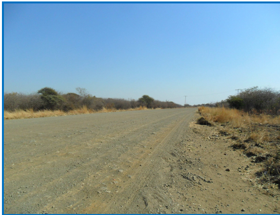
Plate 28: View of Road 108 (direction west)
