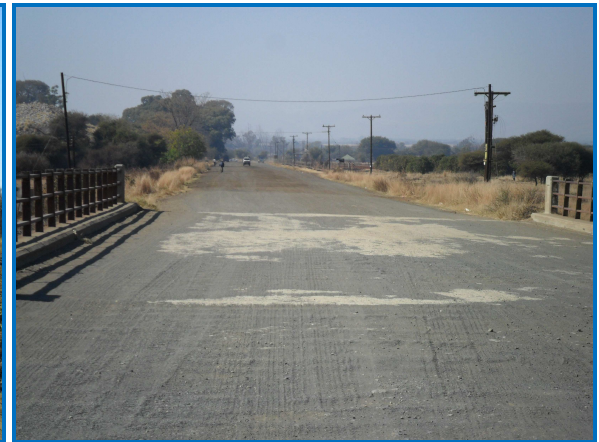
Plate 29: View of Road 108 (direction east)
