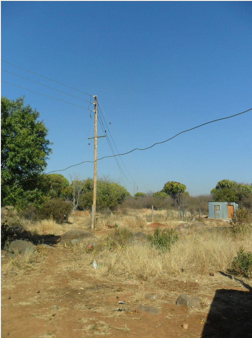
Plate 19: View of existing powerline traversing central portion of development area
