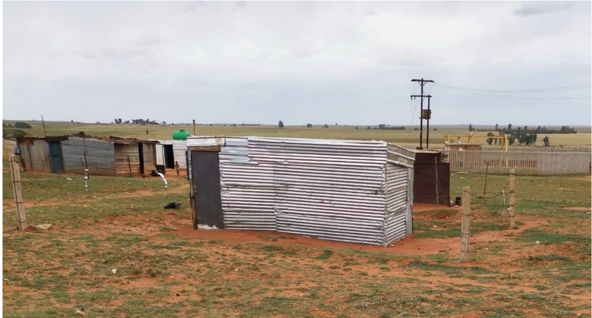
Photo 4: Informal dwellings on site
