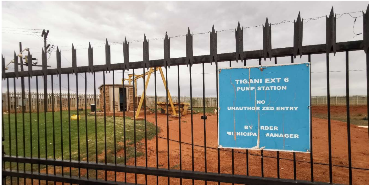
Photo 1: Existing Pump Station on Site (Tigane X8)
