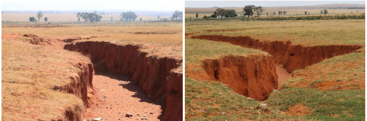
Photo 6: Erosion present on site
