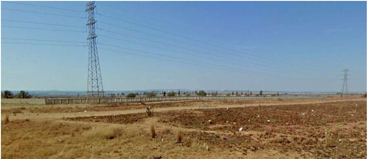
Photo 3: Eskom powerline that runs across site
