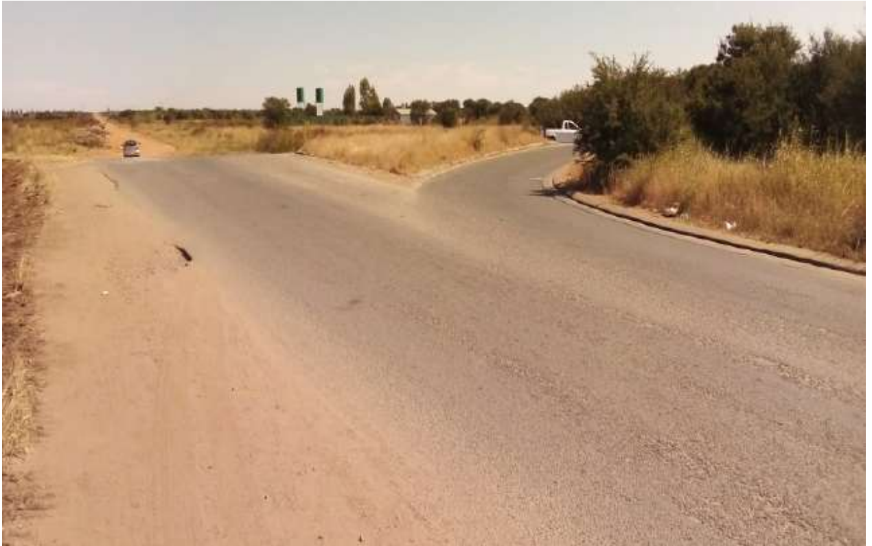
Photo 5: Photo of Road D152 (Swartkoppies Road)
