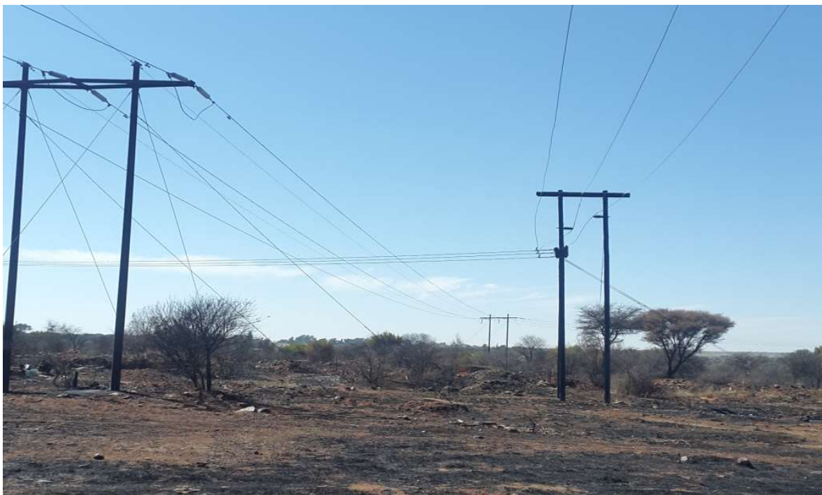
Photo 12: View of existing 88kV overhead line
