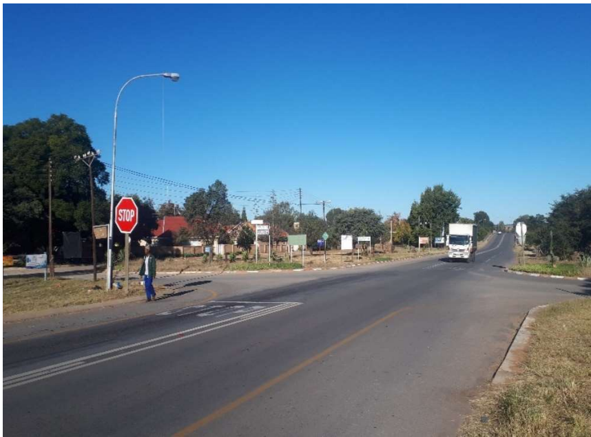
Photo 11: Photo of Road R34 entering Schweizer Reneke from the west
