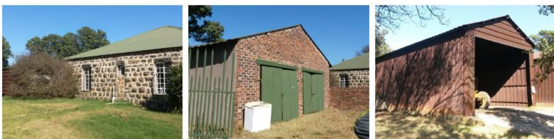
Figure 3: Existing Buildings on Site
