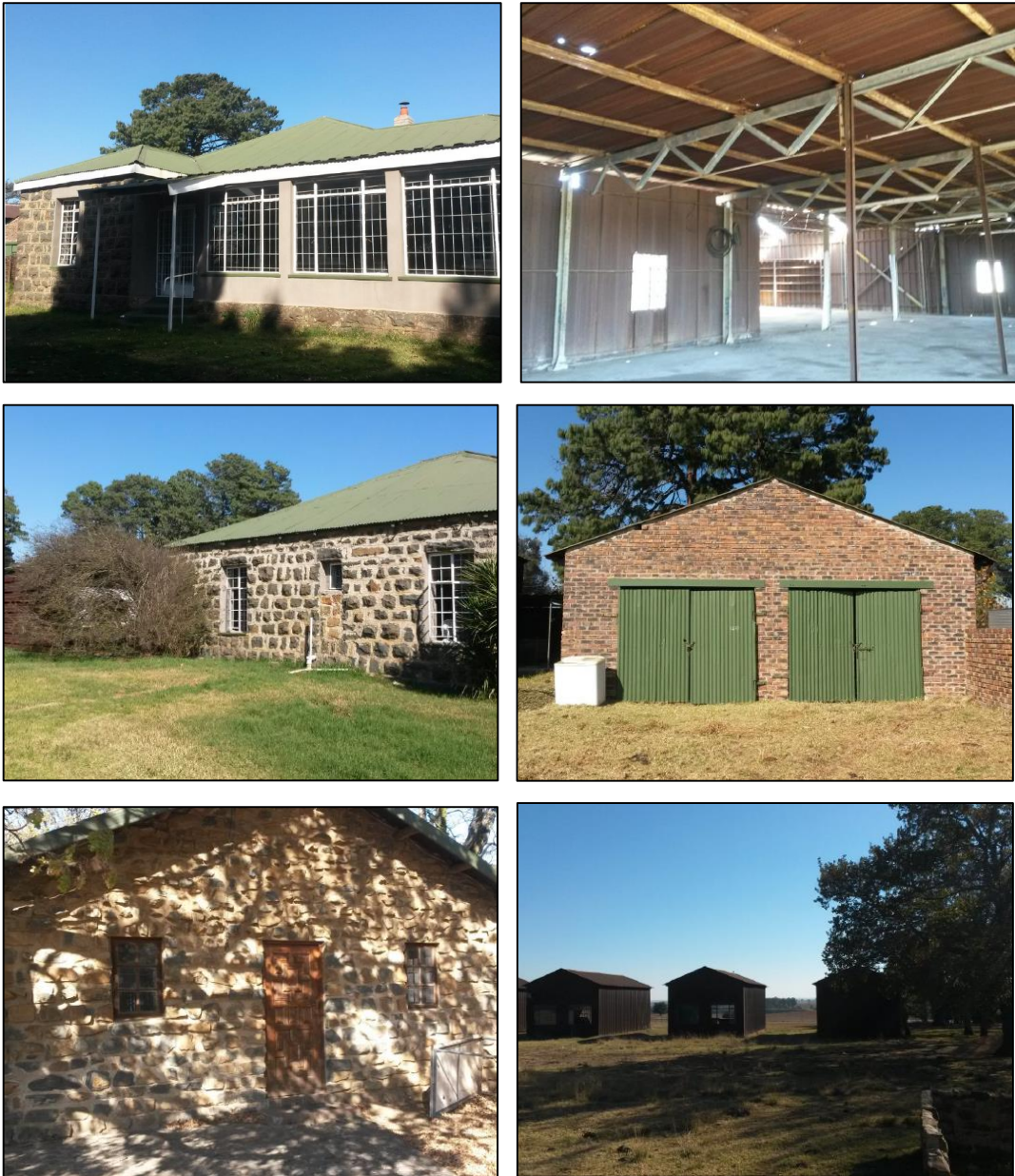
Figure 9: Existing Buildings on Site
