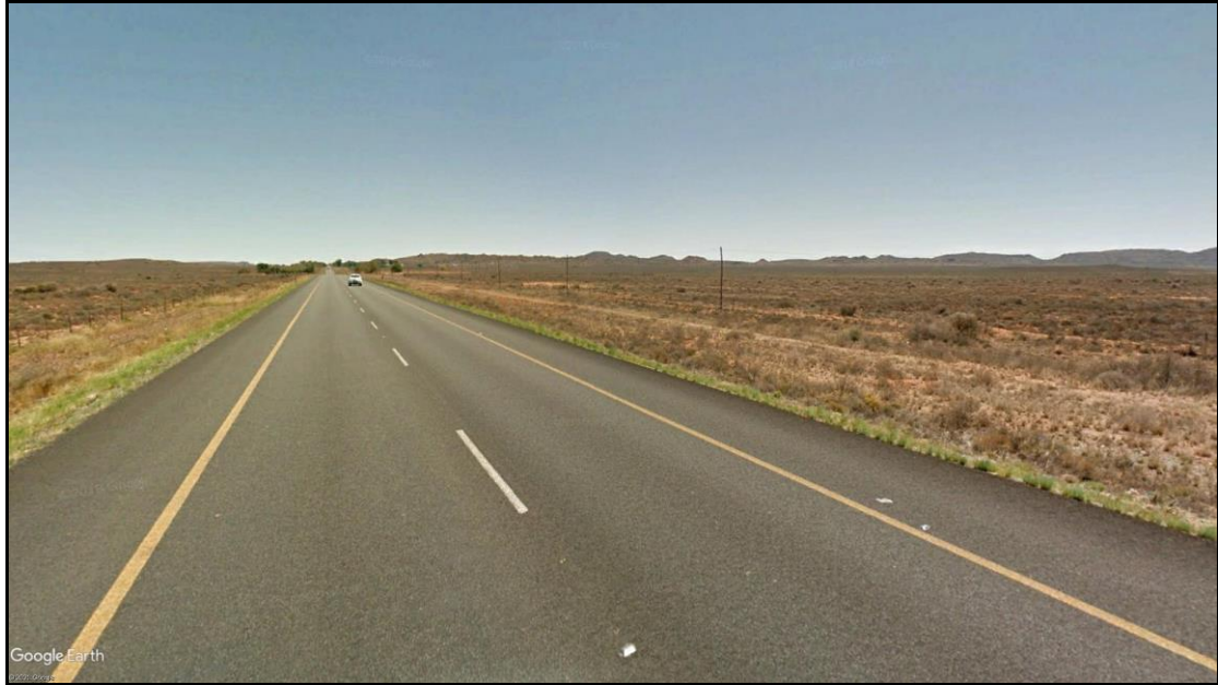
Figure 3: The N1 national road traversing the study area.
