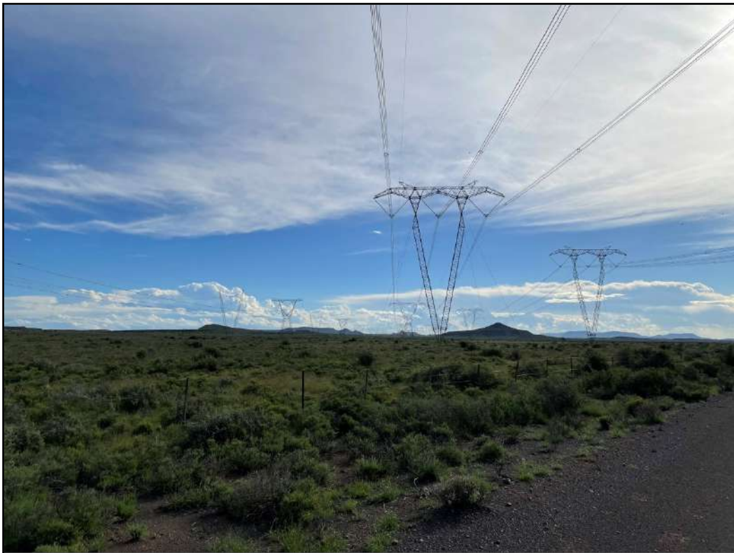
Figure 6: Existing power lines crossing the Hutchinson secondary road (looking to the south-west).
