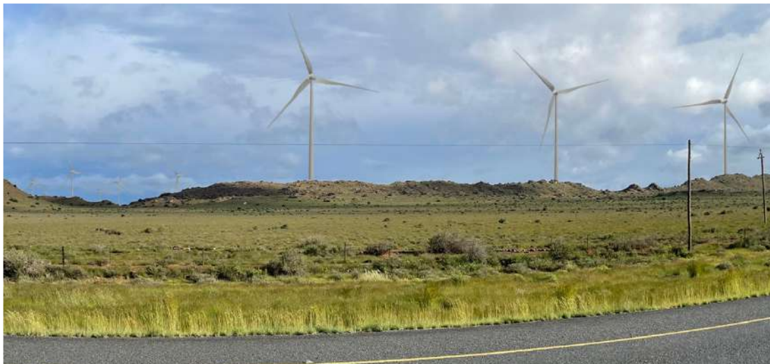
Figure 44: Three of the eight wind turbines located on the Bakenskop ridge.
