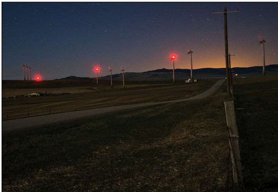
Figure 42: Aircraft warning lights fitted to the wind turbine hubs (Source: http://www.pinchercreekecho.com/2015/04/29/md-of-pincher-creek-takes-on-wind-turbine-lights. )
