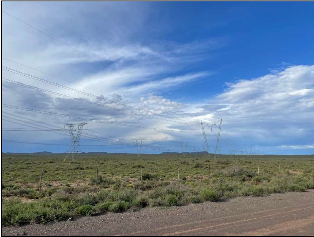
Figure 5: Existing power lines traversing north-west of the proposed WEF site.
