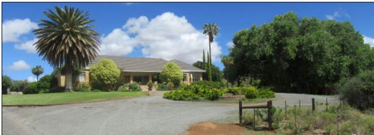
Photograph 3.11: Rondawel farmstead, located near the N1- Hutchinson Road intersection
