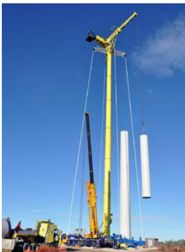
Figure 2-6: Example - Cranes at work
