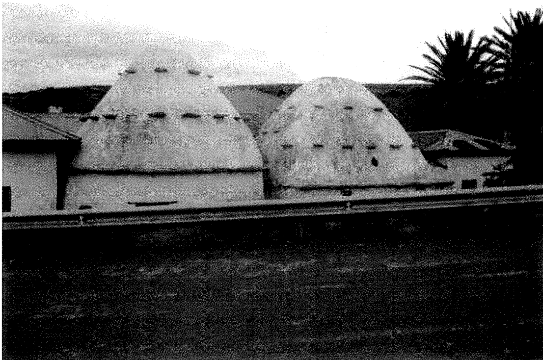
Figure 24. These corbelled dwellings, declared national monuments' are the two most important buildings that may be affected by heavy duty transport vehicle. The main road literally passes within four meters of the stone constructions.
