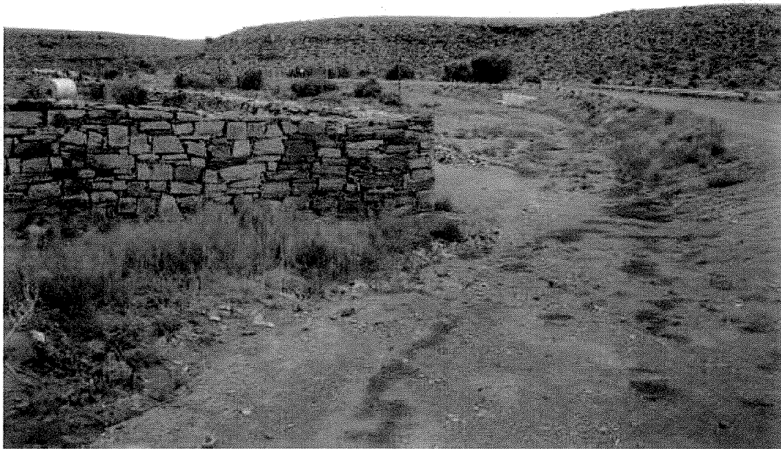
Figure 23. A dry stone walled sheep byre directly adjacent to one of the proposed routes along which heavy duty transport vehicles will be possible used.
