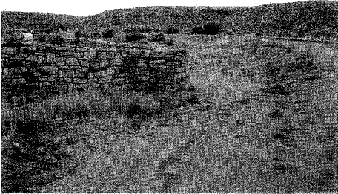
Figure 23. A dry stone walled sheep byre directly adjacent to one of the proposed routes along which heavy duty transport vehicles will be possible used.
