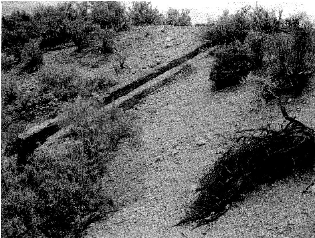
Figure 8. The research area is located within the walls of an old dam.
