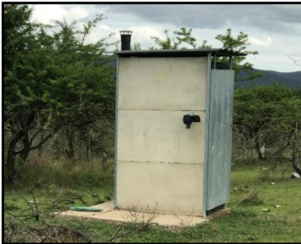
Figure 9.24: Example of pit latrine.
