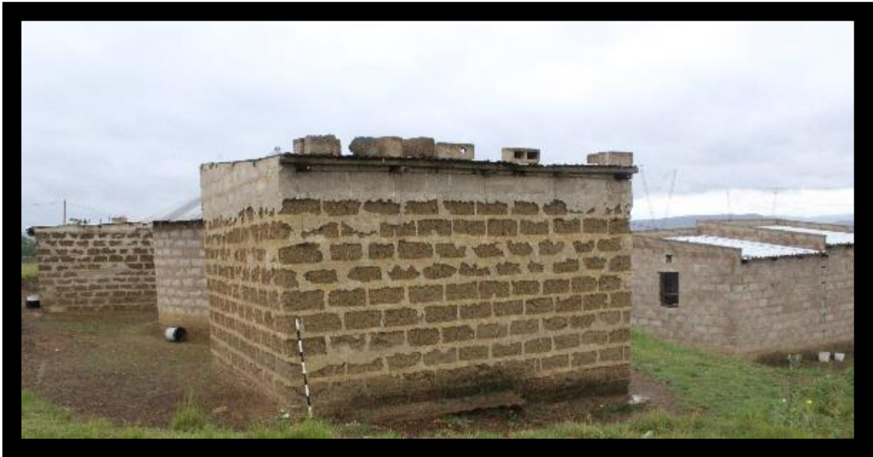
Figure 9.12: Compound with multiple brick flat roof houses
