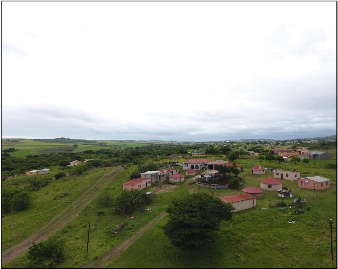
Photo 6.1: An example of a traditional Zulu homestead or uMuzi
