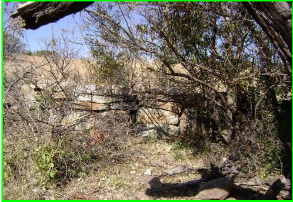
Figure 9: A section of stone wall which was noticed on the north facing bottom slope
