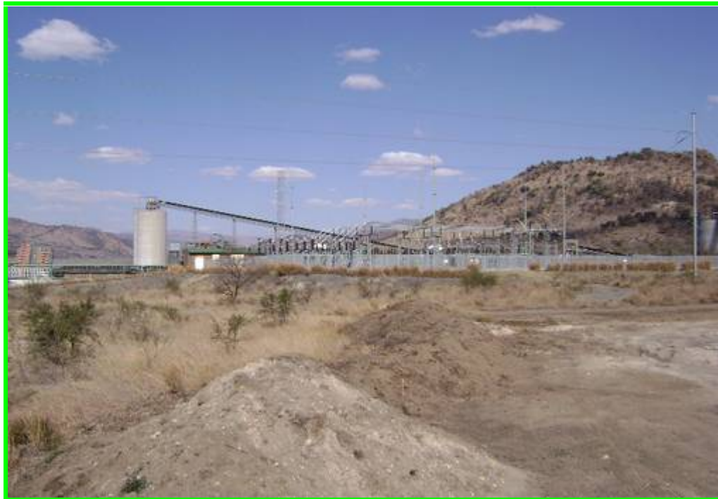
Figure 6: View of the Anglo platinum Mototolo joint venture mine where Der Brochen substation is situated.
