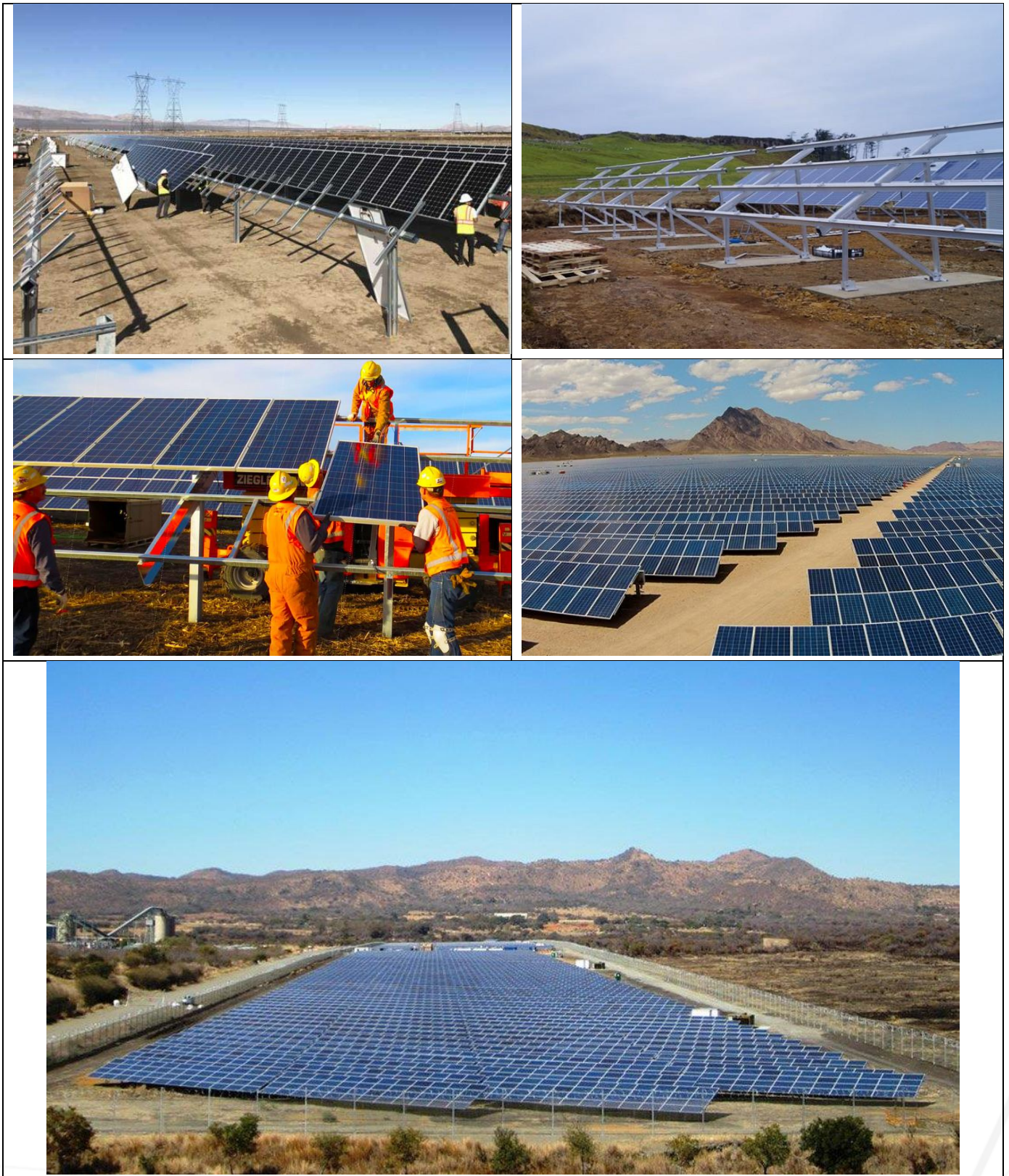
Figure 2.5 Photographs of the construction phase of a solar facility similar to the Middelvlei Solar PV Project (Source: https://medium.com/@solar.dao/how-to-build-pv-solar-plant-6c9f6a01020f ; https://www.shutterstock.com/video/clip-1028794-workers-mounting-panels-on-solar-power-plant-
