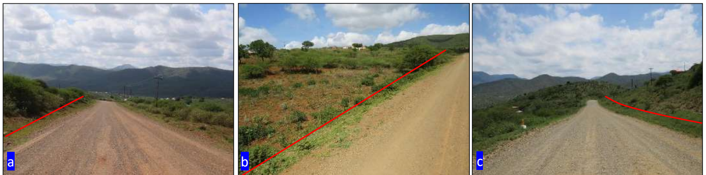
Figure 37: (a): A section of road that the pipe will be laid parallel to. (b): Image showing section of road running parallel to the proposed pipeline; (c): A section of the proposed pipeline (red line) route.
