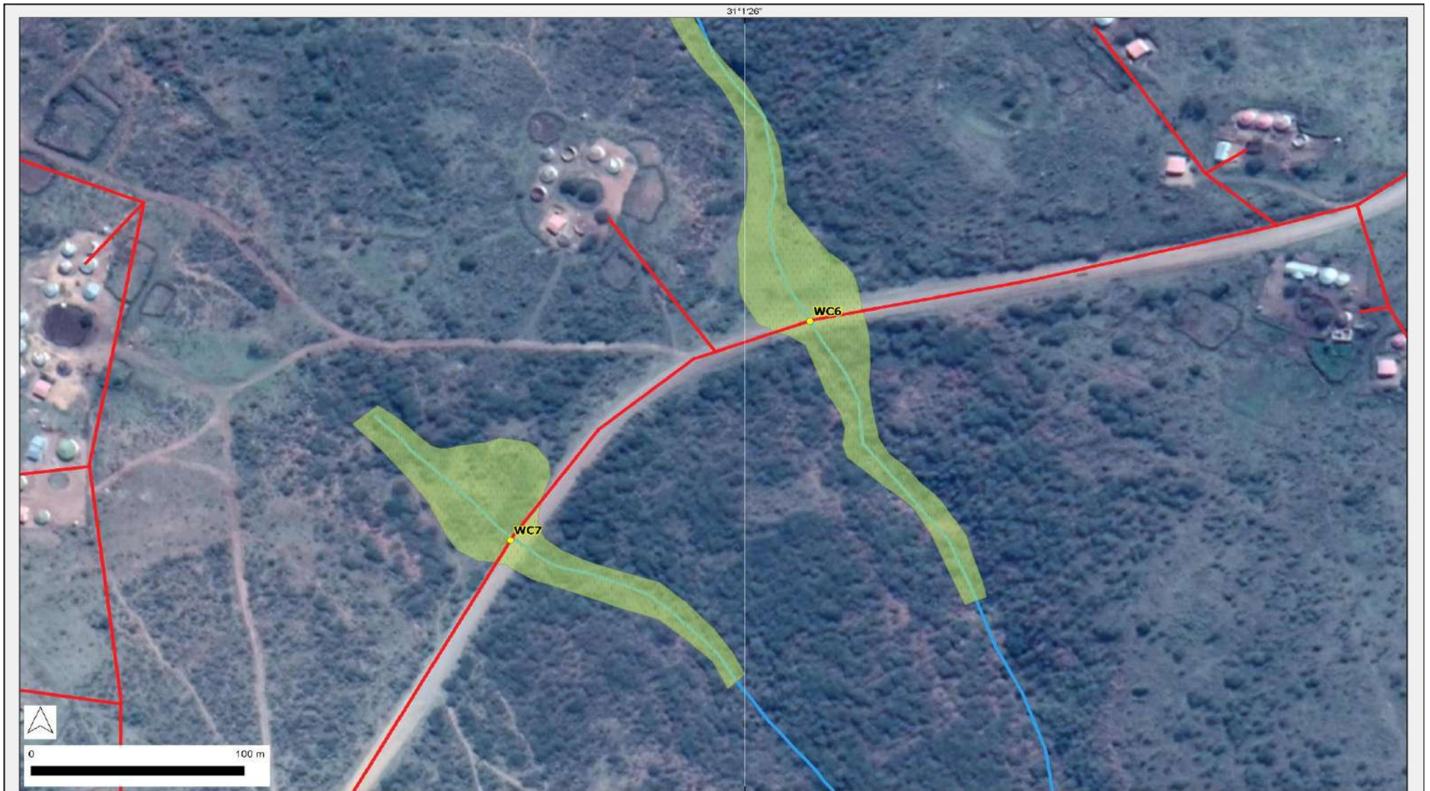
Figure 10: Aerial Photograph Showing the location of WC6 (28°50'14.03"S; 31°1'27.53"E) and WC7 (28°50'17.72"S; 31°1'22.33"E). QGIS, version 3.4.
