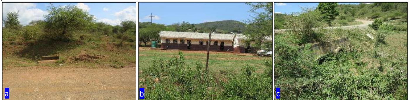
Figure 38: (a): Existing stormwater infrastructure associated with the road running parallel to the proposed pipeline; (b): School located in close proximity to WC18; (c): Existing stormwater infrastructure which the proposed pipeline will be
