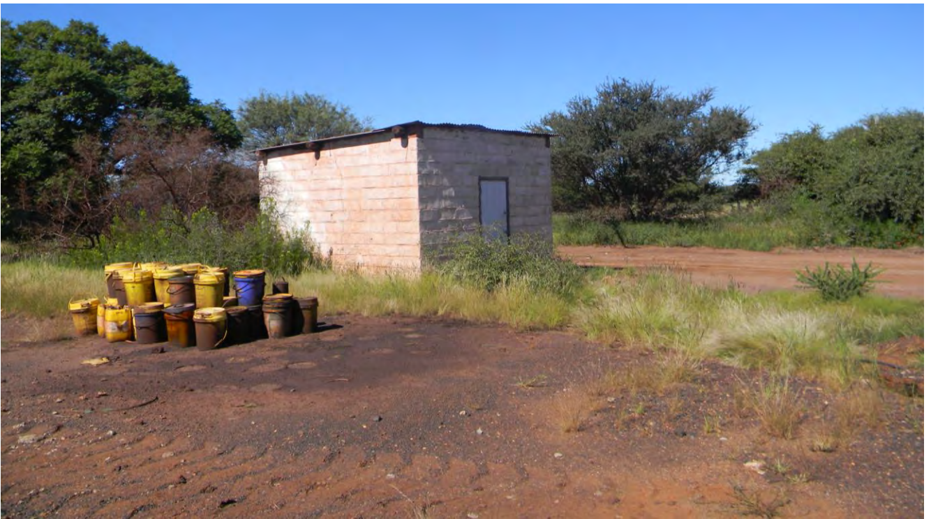
Plate 30: Photo 30: View of the proposed mining right application site (Photograph © by Author 2022)
