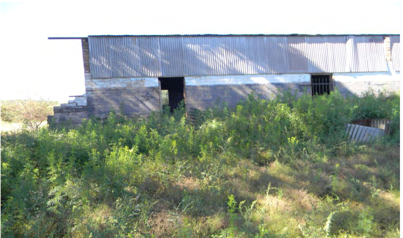
Plate 44: Photo 44: View of the proposed mining right application site (Photograph © by Author 2022)
