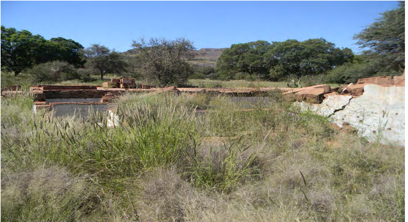
Plate 33: Photo 33: View of the proposed mining right application site (Photograph © by Author 2022)
