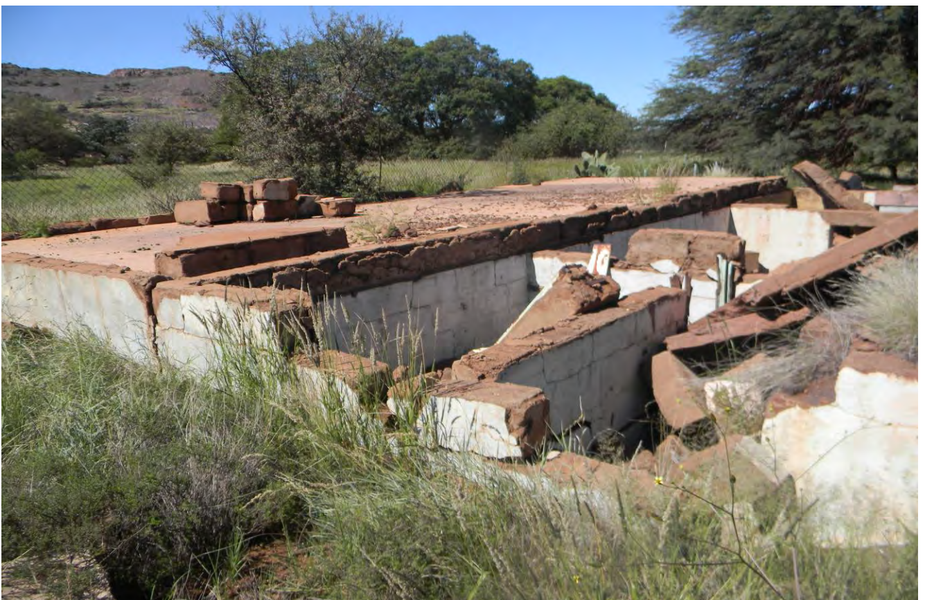
Plate 34: Photo 34: View of the proposed mining right application site (Photograph © by Author 2022)
