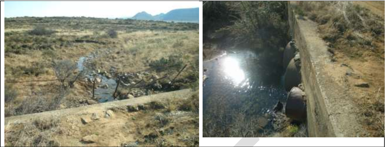
Figure 2.8. Access road bridge over the Wolwekop Stream
