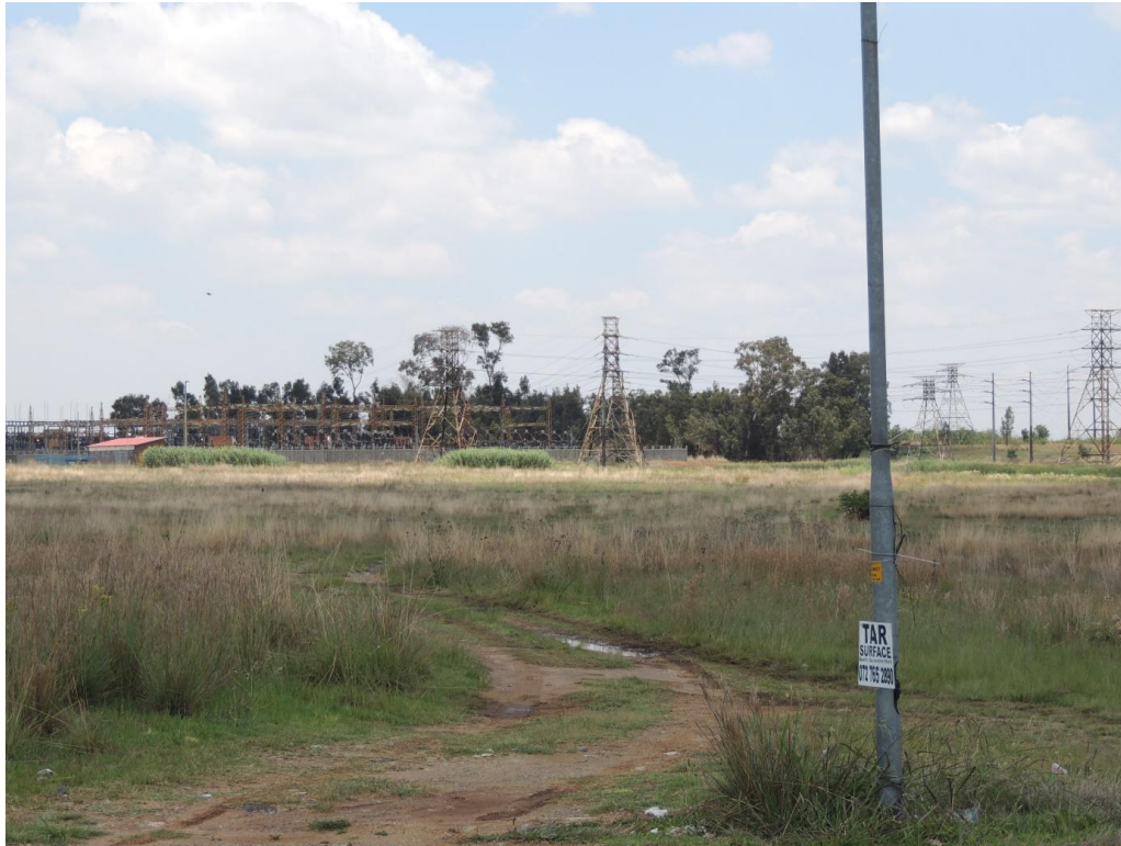
Figure 17: View of the Van Eck substation on site
