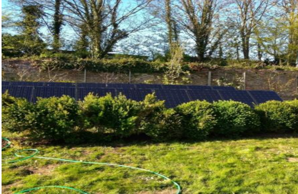
Plate 19, PV array screened by low vegetation. It is possible to screen a PV array from close viewpoints at a similar level to ground level within the array.
