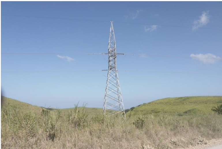
Plate 2, Eskom 132kV Lattice Tower 25-28m high. 132kV structures will be slightly higher than existing and will follow the existing power line servitude.
