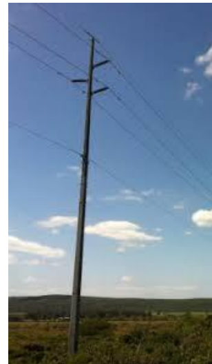
Plate 3, Eskom 132kV Monopole.
