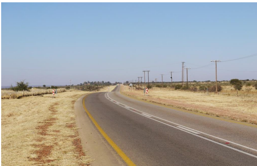
Plate 16, Existing MV overhead cables on the western side
