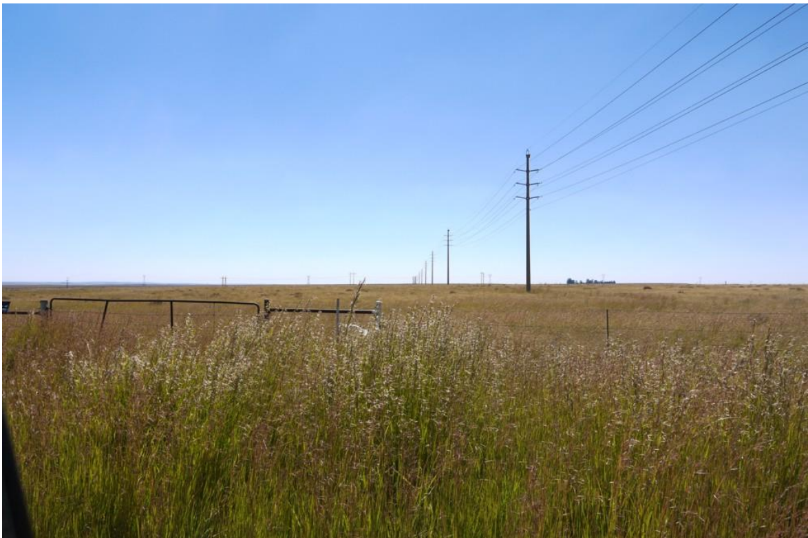
Plate 24, View of a 132kV overhead power line similar line to that proposed. Note pylons on the horizon (approx 2.5km distance) are just visible.
