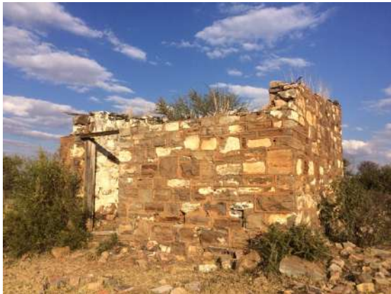
Figure 30 - Single room stonewalled structure at site 019.
