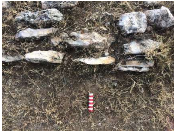
Figure 29 - Stone exterior walling and additional foundations located adjacent to the standing structure.
