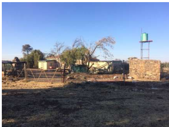
Figure 50 - Mixed-use settlement adjacent to the N18 and opposite the Tiger Kloof School. Construction is primarily stone, with the recent addition of newer materials due its current occupation.
