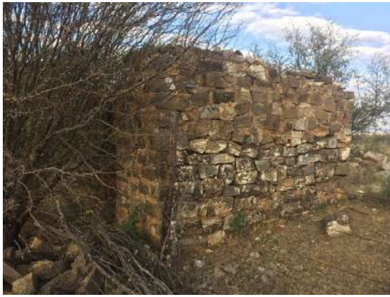
Figure 28 - Single room stonewalled structure at site 018.
