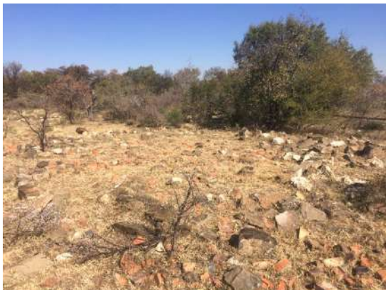
Figure 42 - Poorly preserved structure at site 028, showing presence of bricks, stone and cement.
