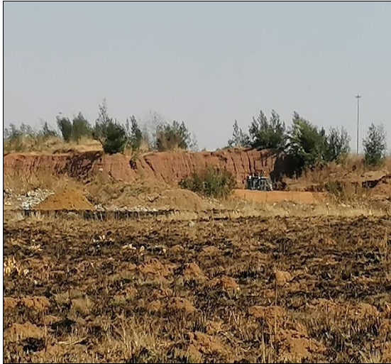
Illegal quarrying on site
