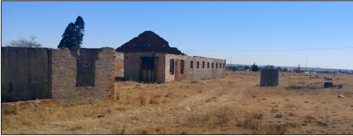
Figure 12: View towards the northwest of the main dairy building (centre) and an outbuilding (left).
