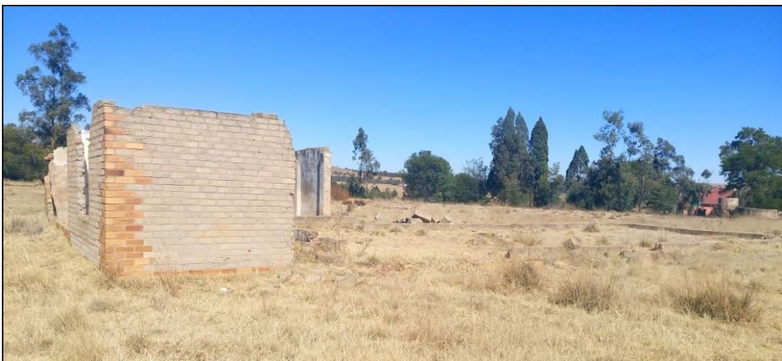
Figure 14: View of the north wall of a second outbuilding to the south of the main dairy building. Some cement foundations are visible to the right. Again, modern bricks are evident.
