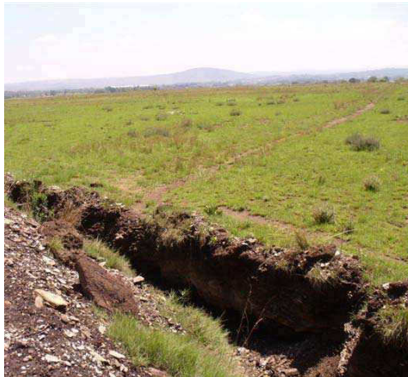
Photo 6: Open trench across grassveld on farm Stukgrond which is a hazardous situation as far as small animals are concerned.
