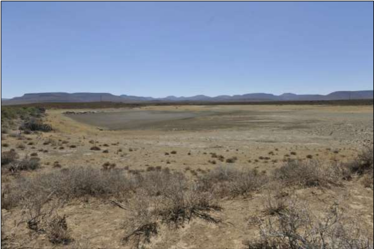
Figure 26: A dam in study area
