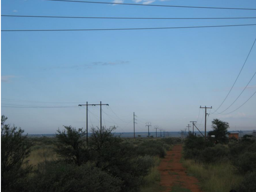
Figure 11: Existing power lines near the Bophirima substation
