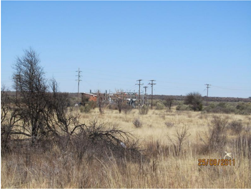
Figure 13: The majority of the areas surrounding the town of Vryburg consists of disturbed grasslands, where the invasion of “thickets” is visible. This photograph was taken in the vicinity of the existing Woodhouse substation.
