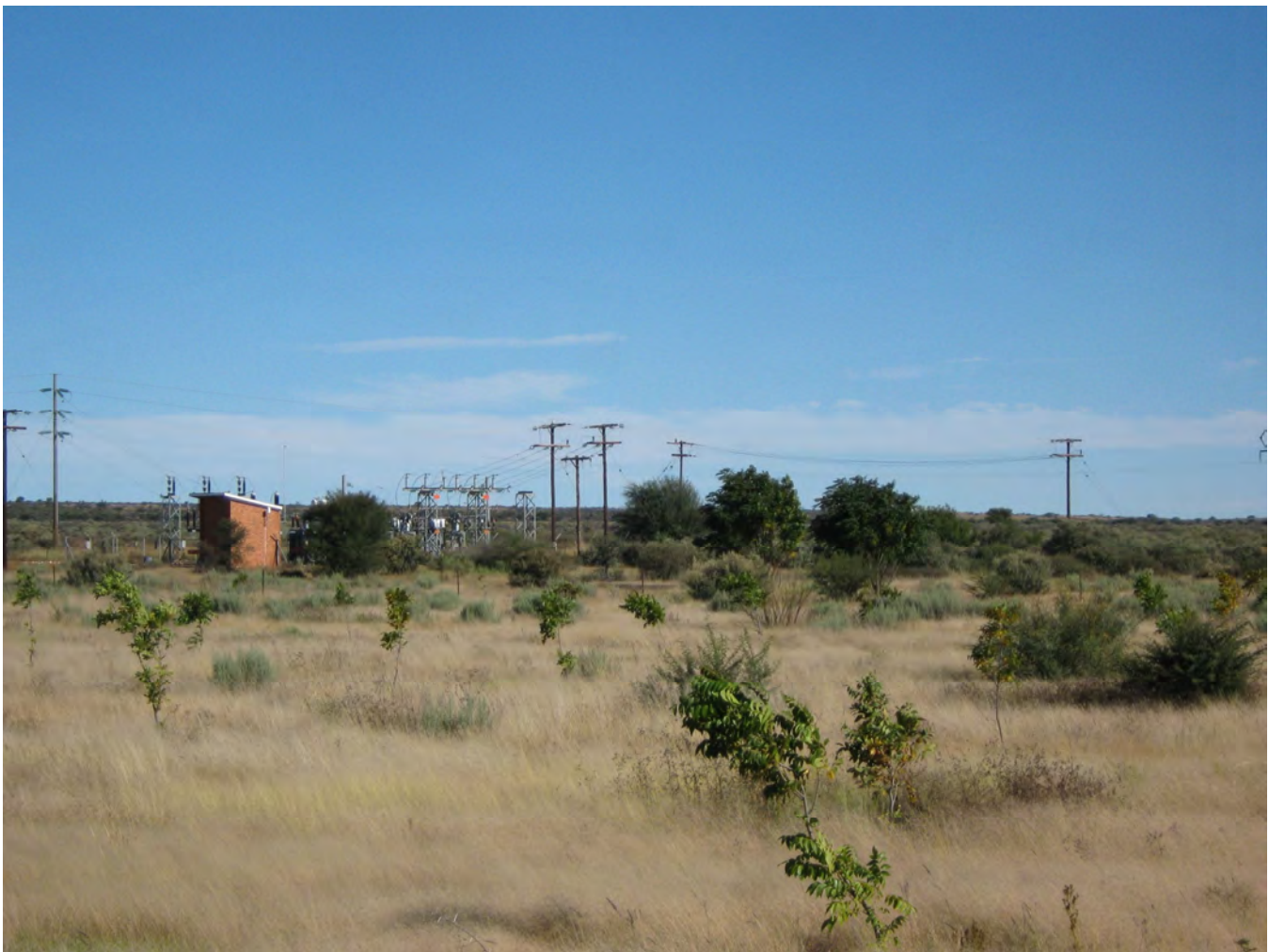
FIGURE 13 – THE EXISTING WOODHOUSE SUBSTATION
