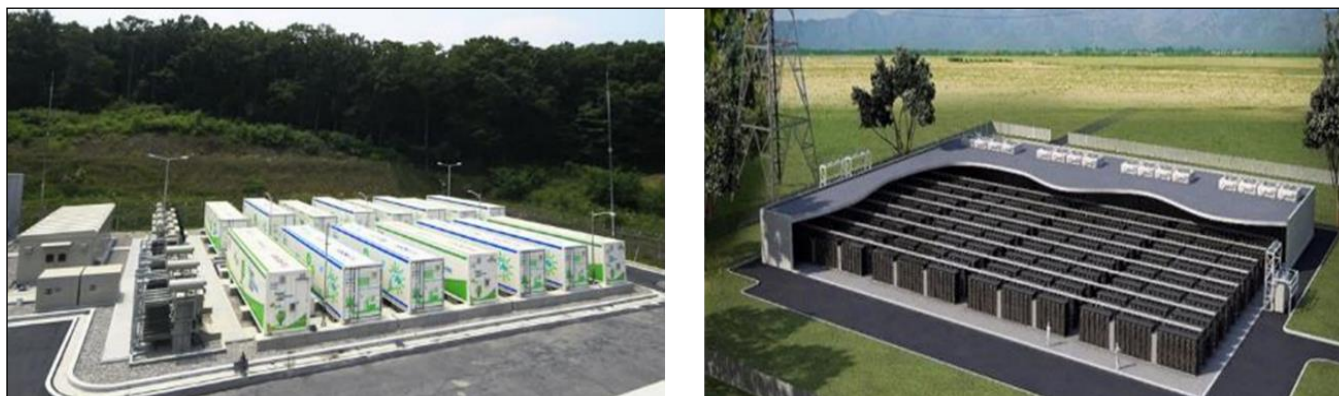
Figure 5. Battery Energy Storage System (BESS)
