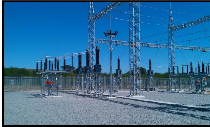
Construction of 132kV Substation
