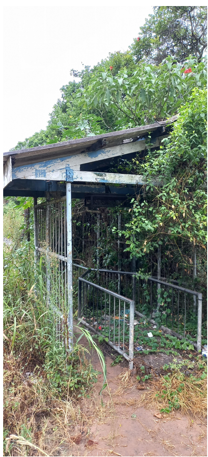
2 - EXISTING ENTRANCE STRUCTURE
