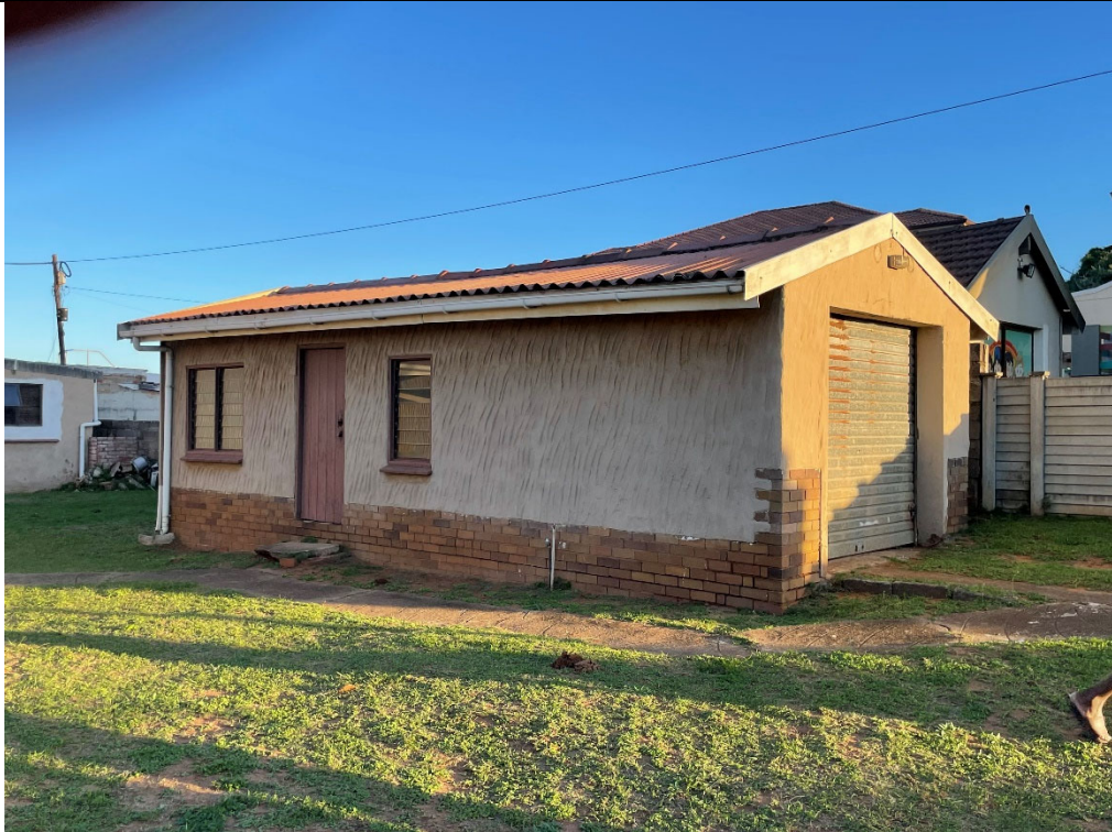
Existing Garage 175 Hillhead Road
