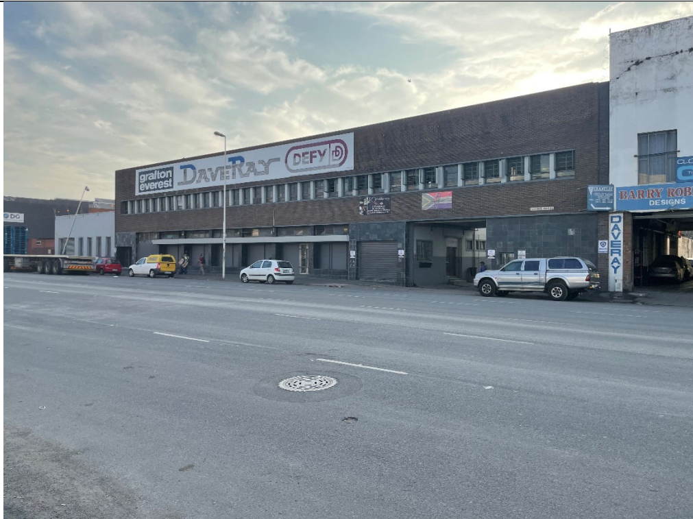
Existing Adjacent Property
