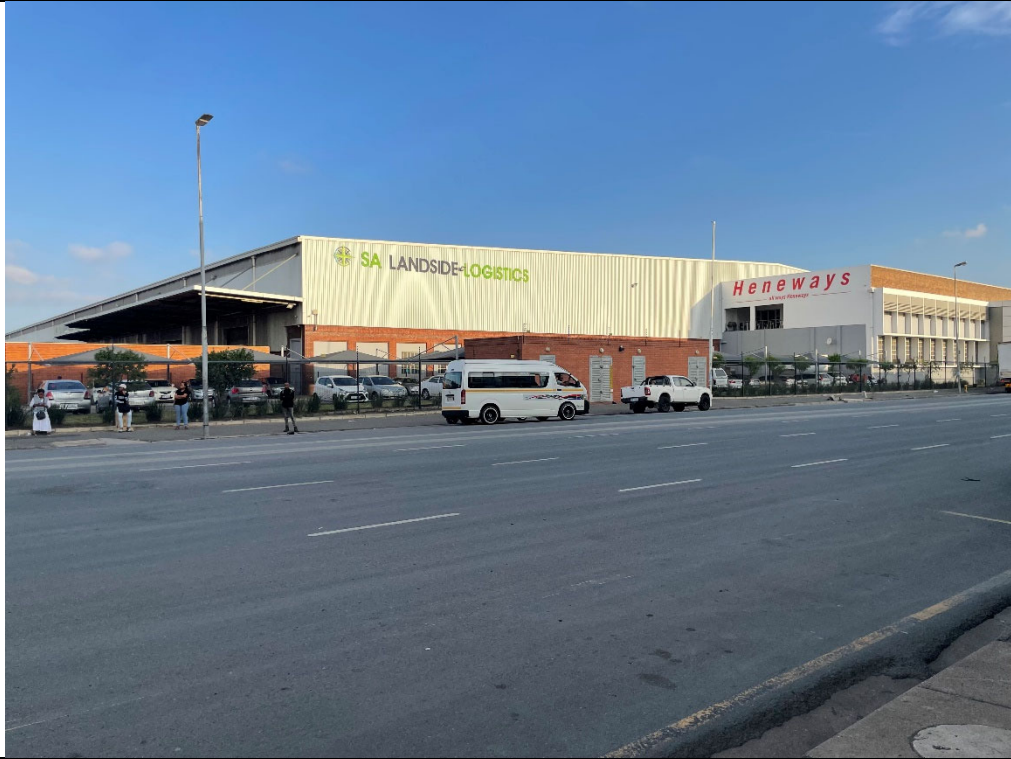
Existing Adjacent Property
