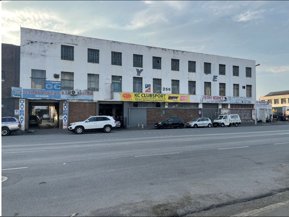
Exterior Photograph No 3 – Sydney Road frontage
