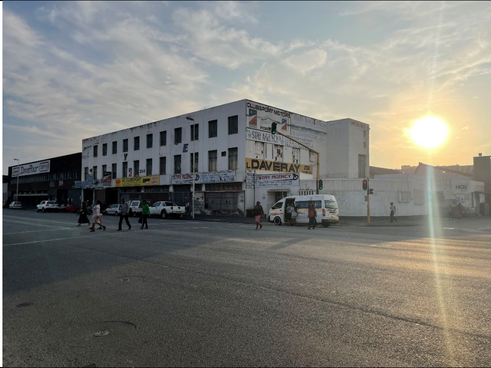
Exterior Photograph No 1 – Corner of Alan Paton & Sydney Road
