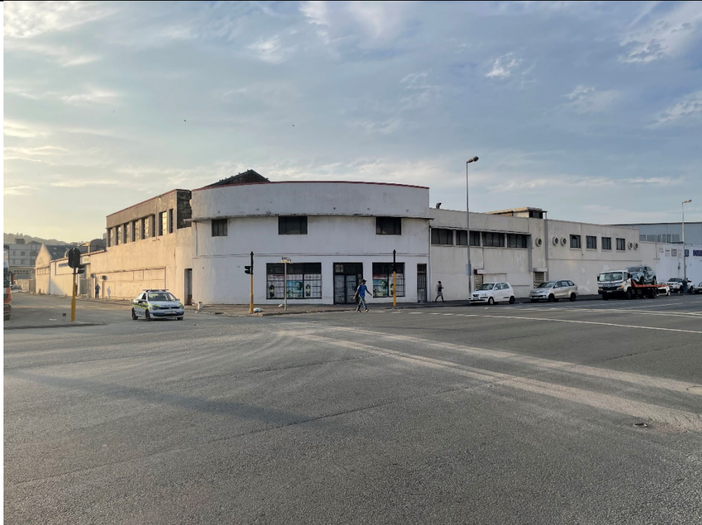
Existing Adjacent Property
