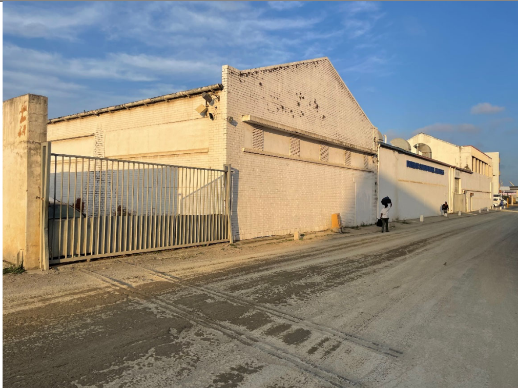
Existing Adjacent Property
