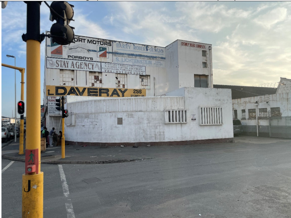
Exterior Photograph No 2 – Corner of Alan Paton & Sydney Road
