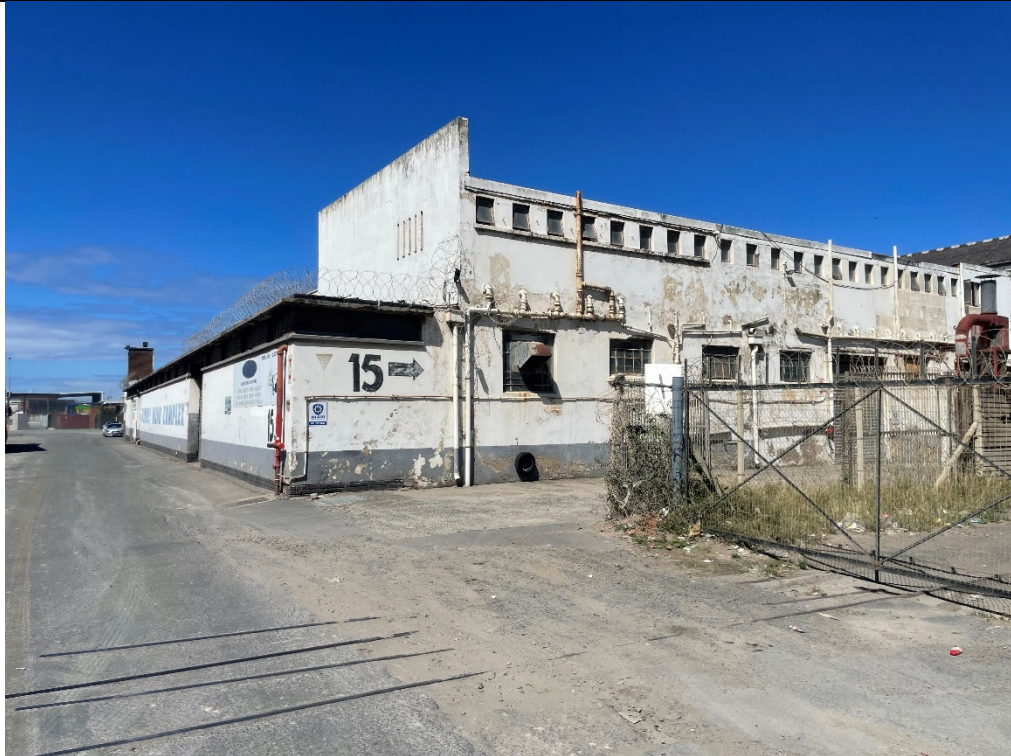
Exterior Photograph No 7 – Alan Paton Road
