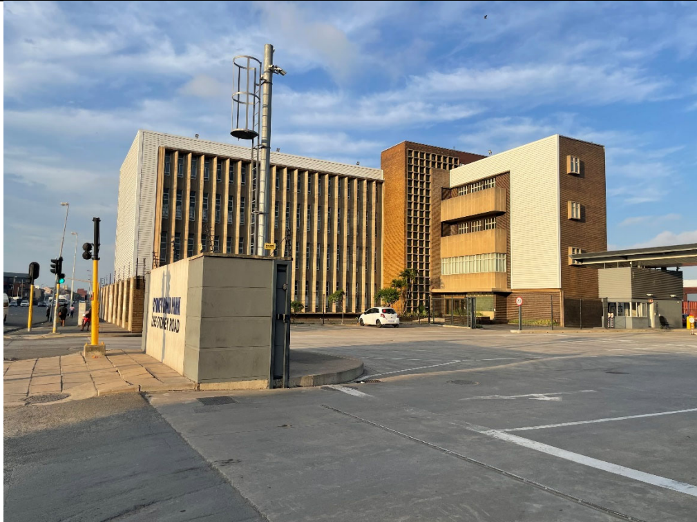
Existing Adjacent Property
