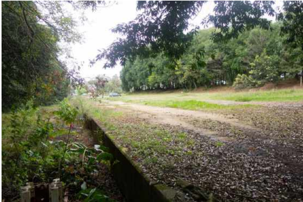
Figure 4. The railway siding, looking to the south. The railway lines (at left but not visible) are still in place. The concrete surfaced platform and adjacent hard surfaces cover most of the property
