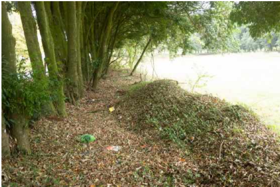
Figure 5. Along the western side of the property adjacent to Hilton Ave, piles of earth and rubble have been pushed to one side
